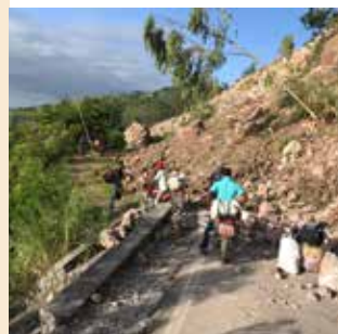
ROADS AND OTHER INFRASTRUCTURE WERE SEVERELY DAMAGED AFTER THE SUMMER 2021 EARTHQUAKE IN HAITI.
