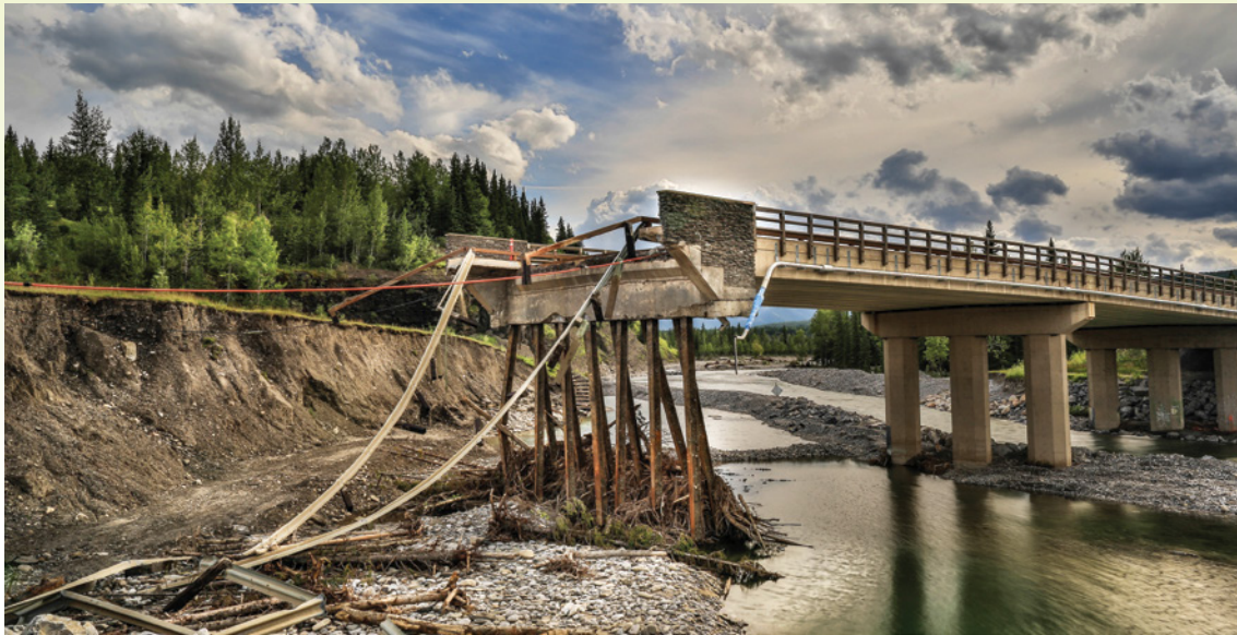
Bridge on the highway to Elbow Falls, Alberta wiped out by rushing flood waters making their way to High River and Calgary in June 2013.
