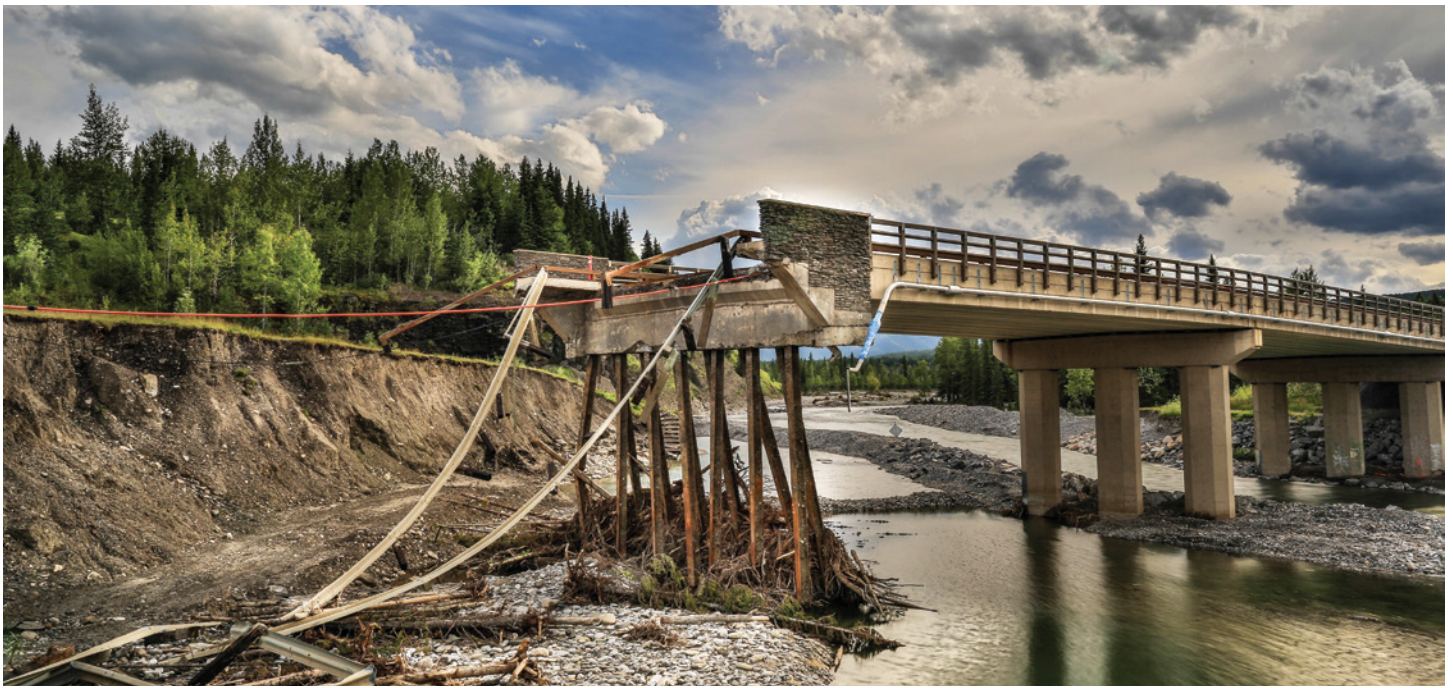
Bridge on the highway to Elbow Falls, Alberta wiped out by rushing flood waters making their way to High River and Calgary in June 2013.
